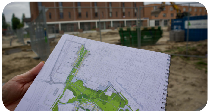
Image: Wielwijk under construction (May 2022), by Caitlin Ball
